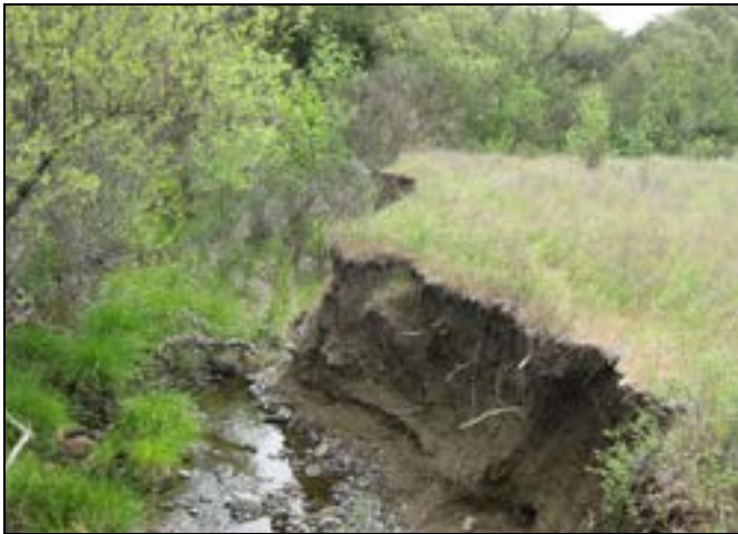
Photo 7. Weeks Creek bank erosion
