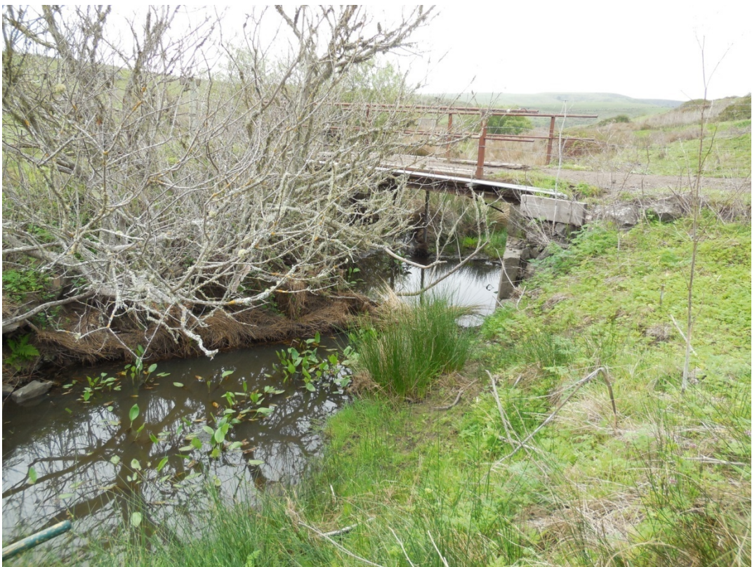
Photo 19. Existing bridge across central creek. (4/15/14)
